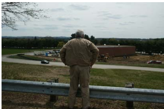
May 2005: Dr. Frank Mevers, NH State Archivist, overlooks early construction site
