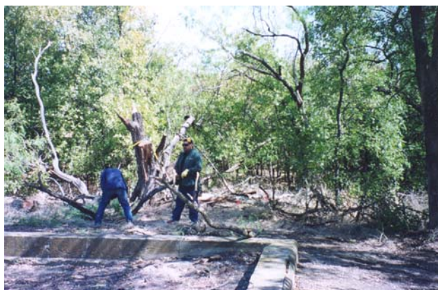
Workers clearing the area around the school foundation, 2005
