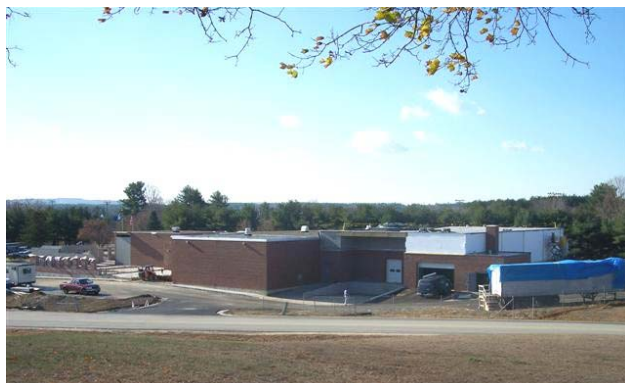
Construction site: November 14, 2005
