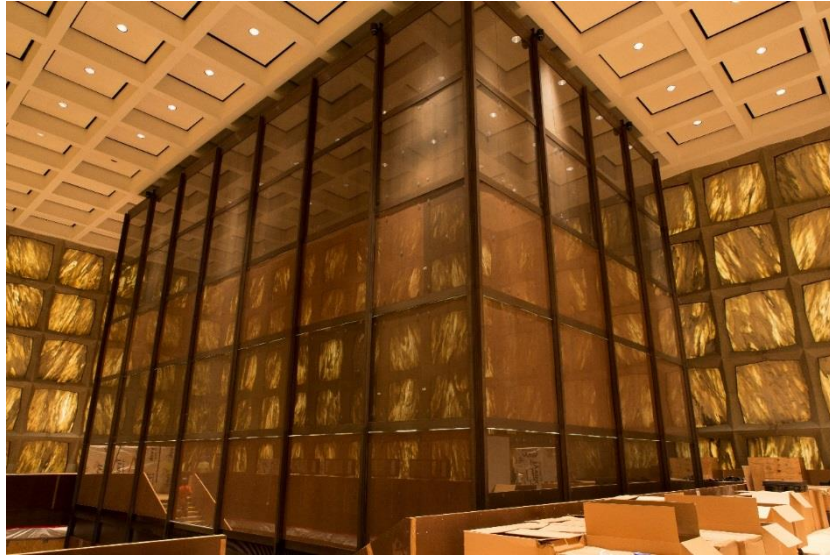
STACK TOWER DURING THE RENOVATION
