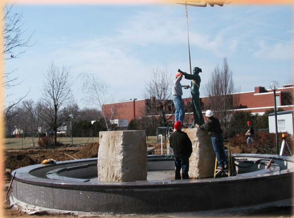
Indiana University South Bend Archives, Crossroads Fountain Installation , March 24, 2003.
