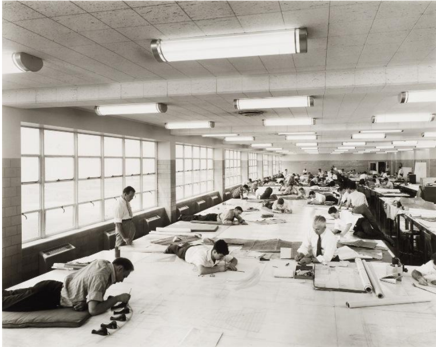
Hedrich-Blessing Photographic Studio, view of the drafting room, 1942, Albert Kahn Associates, Ford Motor Bomber Factory, Willow Run, Michigan, Gift of Federico Bucci © Chicago History Museum.
